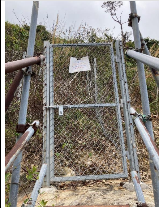
Photo 2 – Current situation of fencing and warning sign
