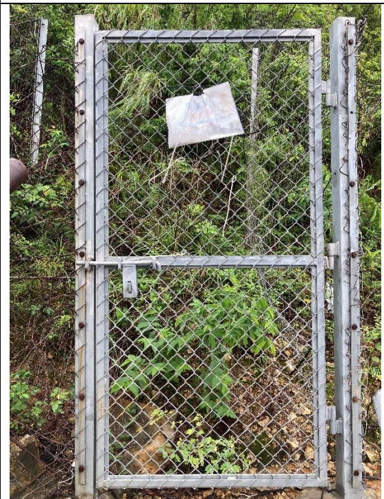
Photo 2 – Fencing and warning sign (As of June 2021)
