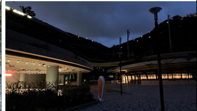
OP06 Responsive Lighting Design – General view of lighting design with appropriate level of lighting to reduce potential impact
