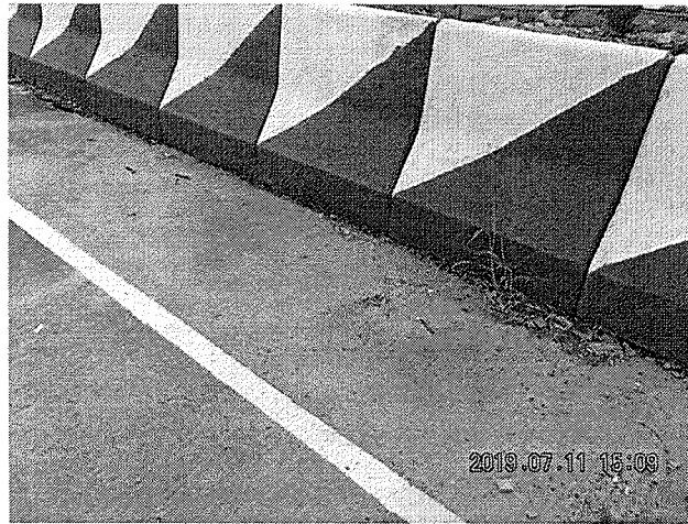
Photo 190711_001(Near Site Exit)(Improved)
