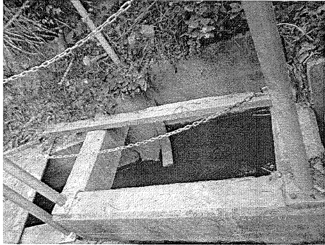
Photo 200324_001 (Near Weighbridge) (Improved)
