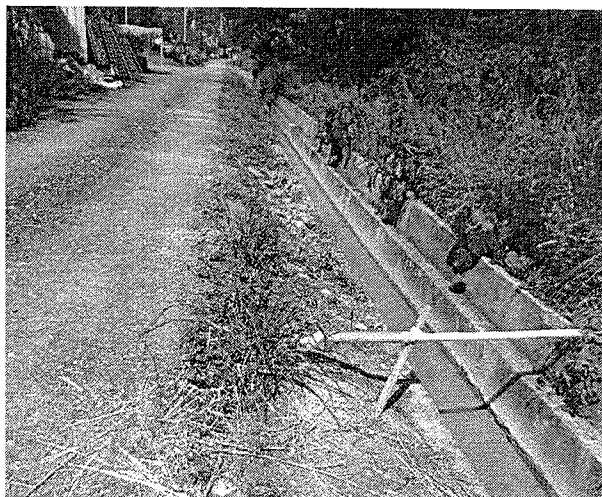
Photo 200429_002 (Near wheel washing facility) (Improved)
