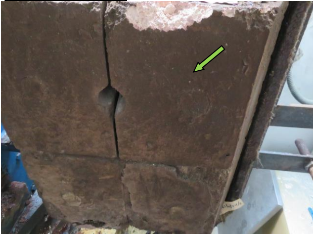
Photo N7. Non-ACM brick to door of incinerator, photo taken at Cage Cleaning Area, 5/F, UPB.
