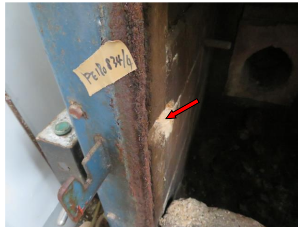
Photo S4. Brick inside incinerator, (PE180834/4), sampled at Cage Cleaning Area, 5/F, UPB, was confirmed as non-ACM.
