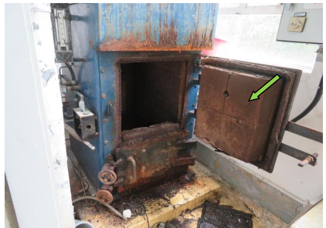
Photo N6. Non-ACM brick to door of incinerator, photo taken at Cage Cleaning Area, 5/F, UPB.
