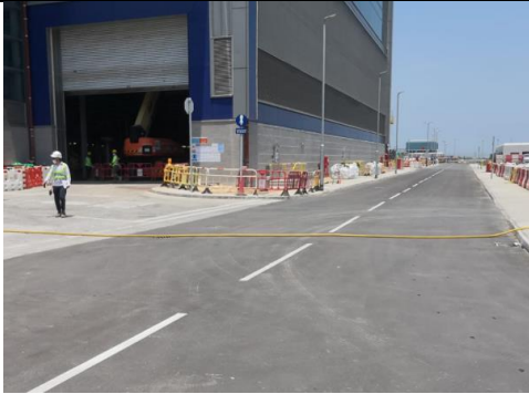
Asphalt pavement was provided to minimize muddy runoff
