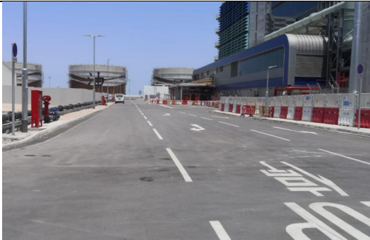
Asphalt pavement was provided to minimize muddy runoff
