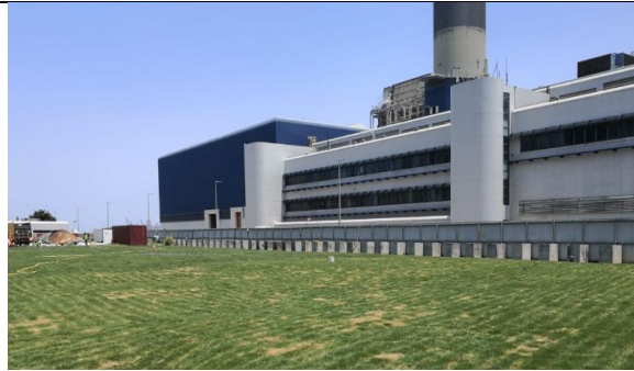
Green Lawn (Grass) has been implemented on site to reduce muddy water runoff
