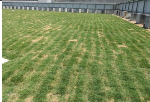
Green Lawn (Grass) has been implemented on site to reduce muddy water runoff
