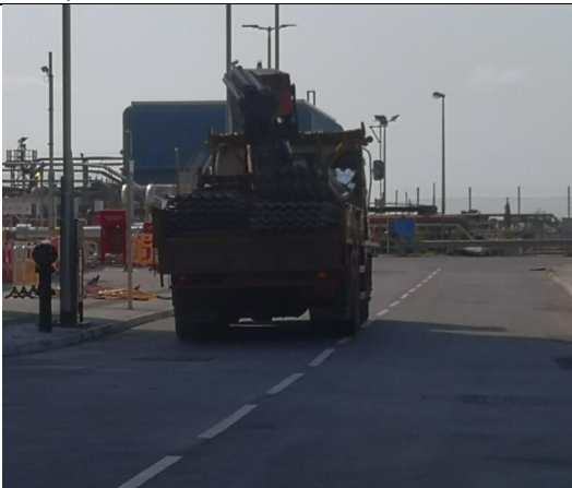
Asphalt pavement was provided to minimize muddy runoff
