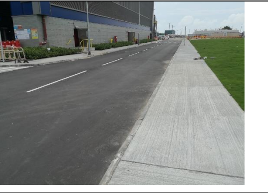
Asphalt pavement has been provided on site to minimize runoff
