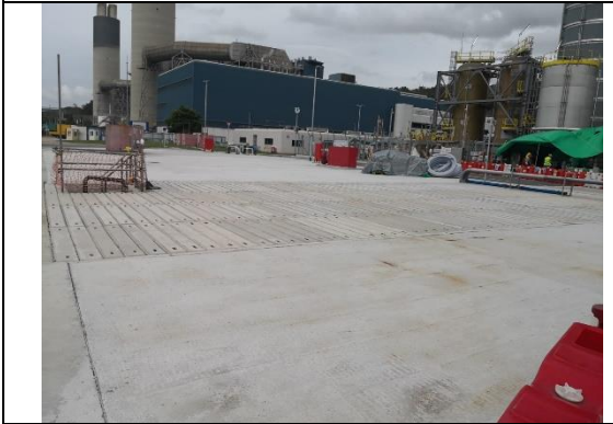
Concrete pavement has been provided on site to minimize runoff
