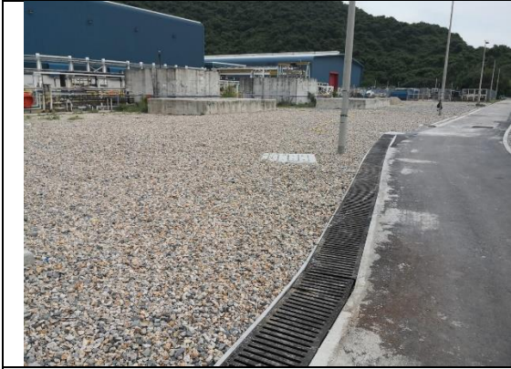
Asphalt pavement has been provided to minimize muddy runoff
