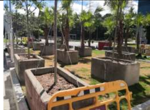
Planter has been built to reduce runoff
