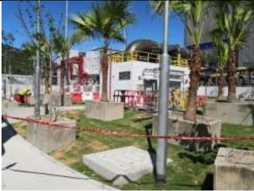
Planter has been built to reduce runoff
