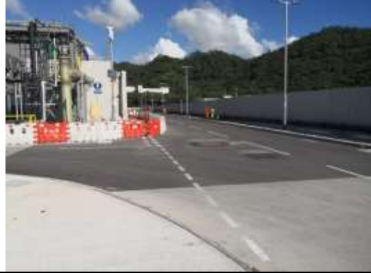
Asphalt pavement has been implemented on site to minimize runoff
