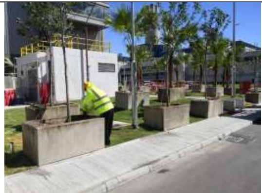
Planter has been built to reduce runoff
