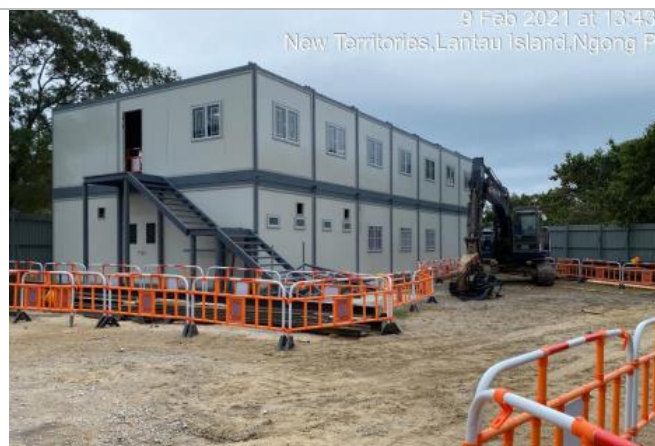
Set up site office
