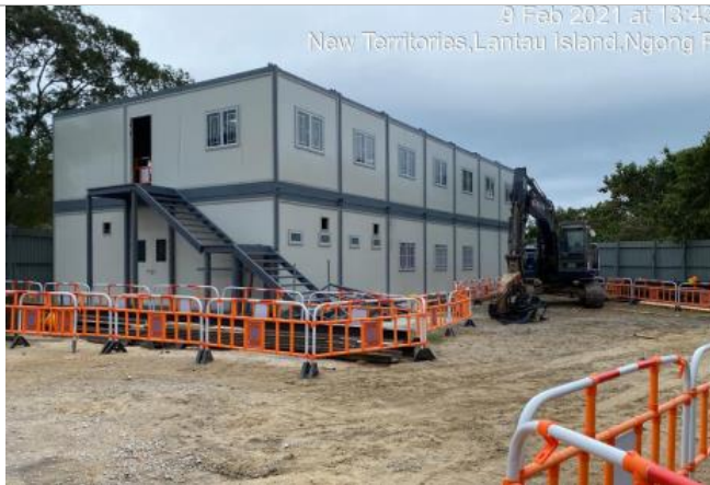
Set up site office
