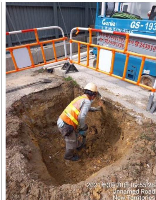
- Excavation of well
