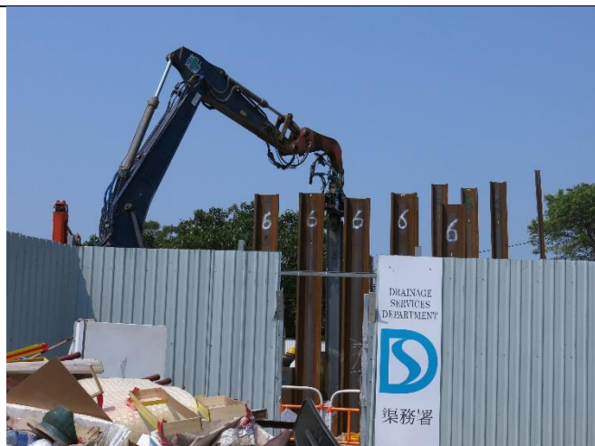
Photo 2: Pile driving works was noted during inspection
