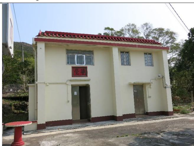
Photo 6: General View of NP-11
