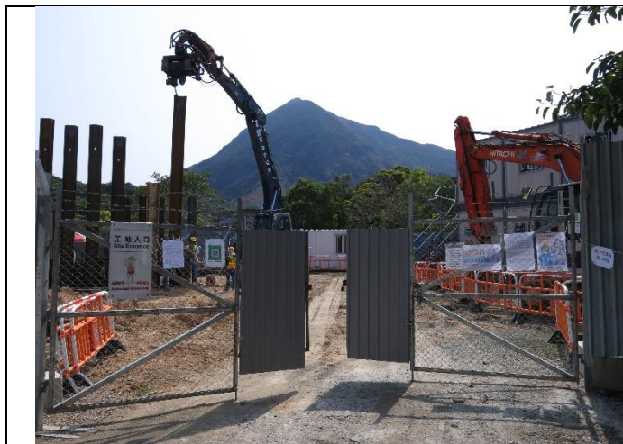
Photo 1: Pile driving works was noted during inspection
