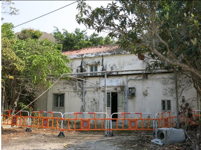
Photo 9: NP-19 has been fenced off in accordance to EM&A Manual
