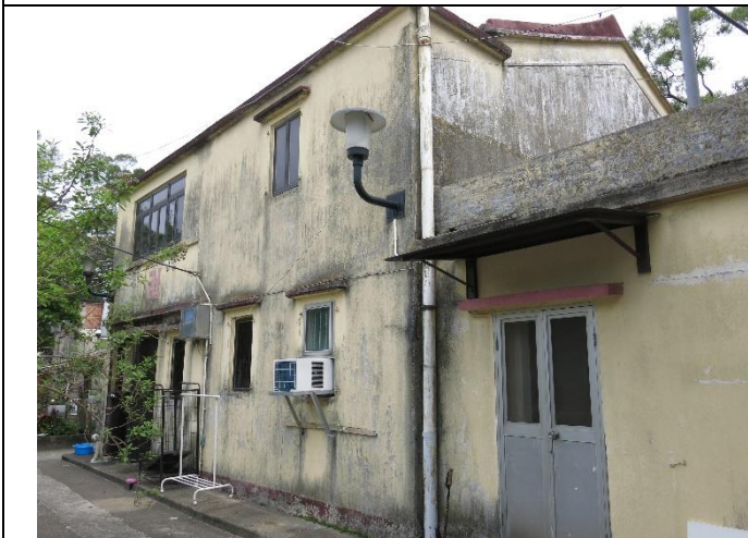
Photo 3: General View of NP-10
