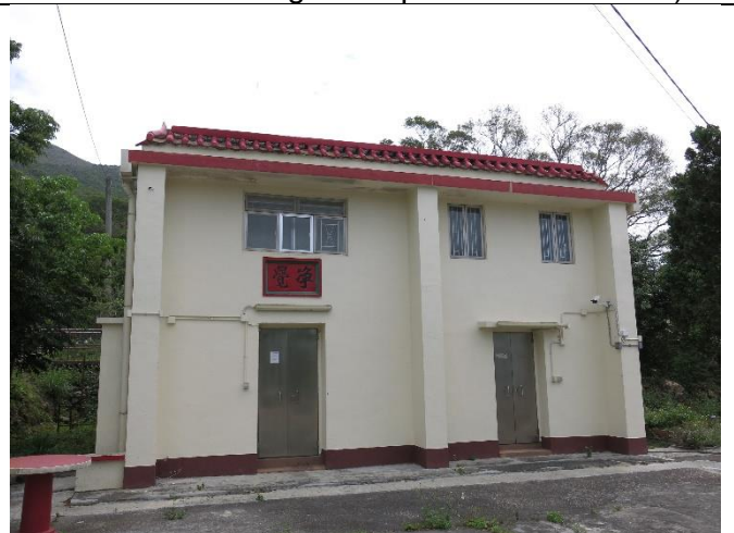
Photo 6: General View of NP-11
