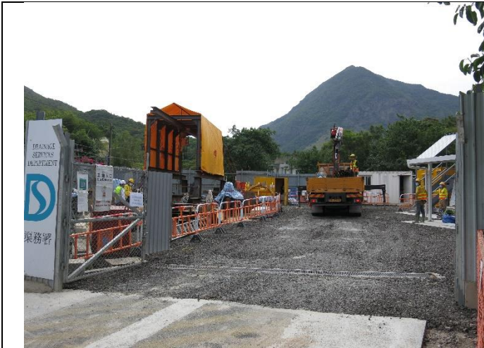
Photo 1: The jacking pit has been constructed
