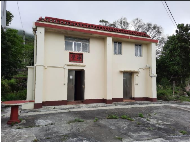
Photo 5: General View of NP-11
