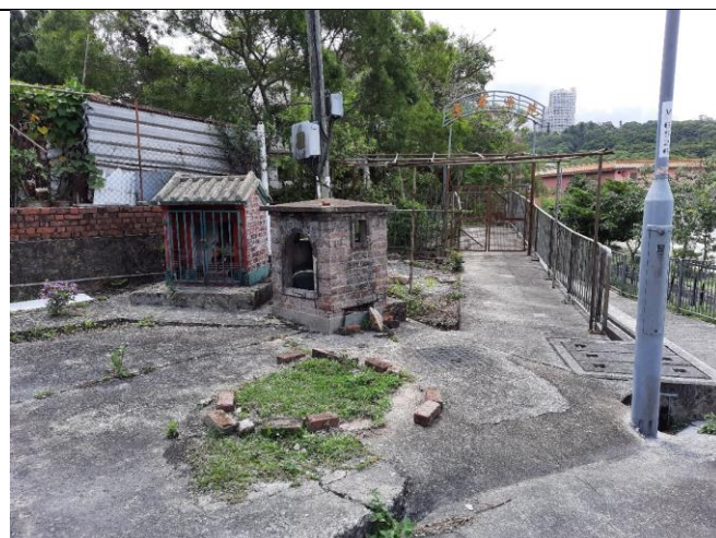
Photo 12: No temporary fence has been erected around NP-26 in mutual agreement with the villagers. No notice to alert the workers has been posted near NP-26.
