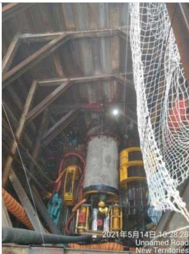
- Trenchless construction by TBM
