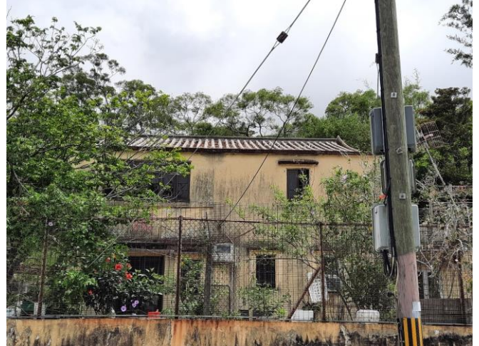
Photo 2: General View of NP-10
