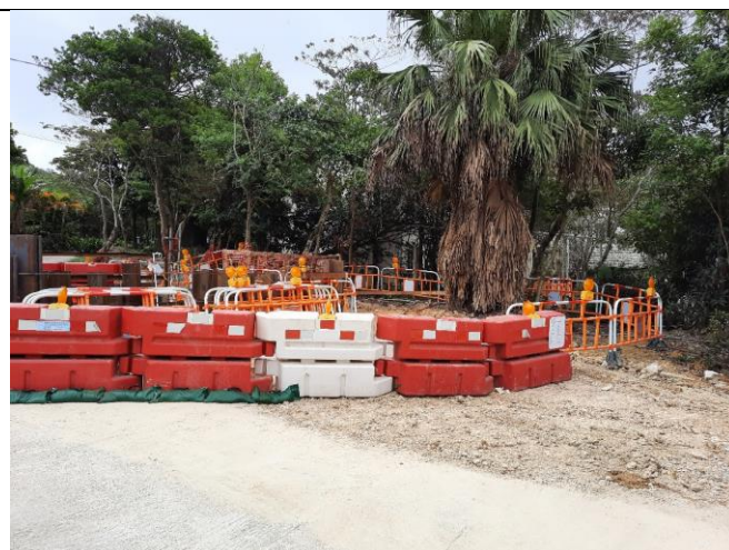
Photo 8: The receiving pit near NP-19 has been constructed.
