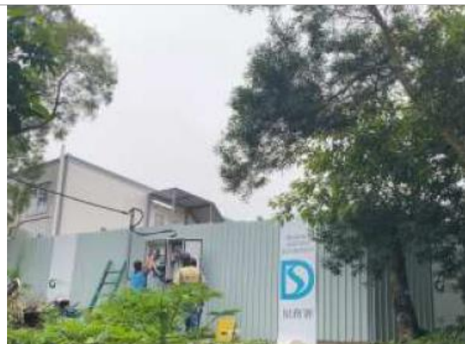
- Set up site office
