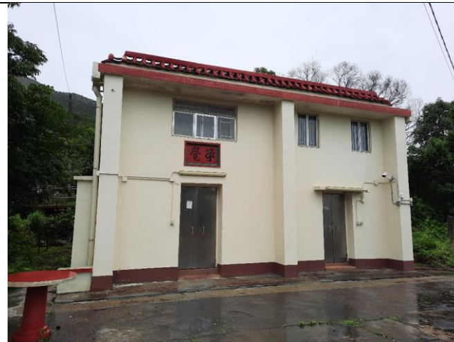
Photo 5: General View of NP-11
