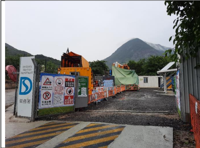
Photo 1: The jacking pit in the opposite of NP-10 has been constructed. Works in progress.
