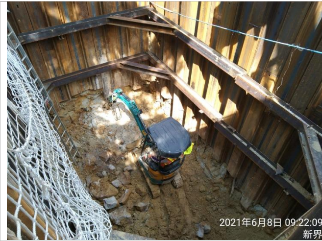
- Excavation Works (Manhole L303)
