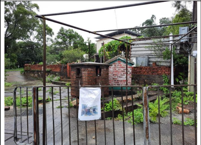
Photo 12: Notice to alert the workers has been posted near NP-26.
