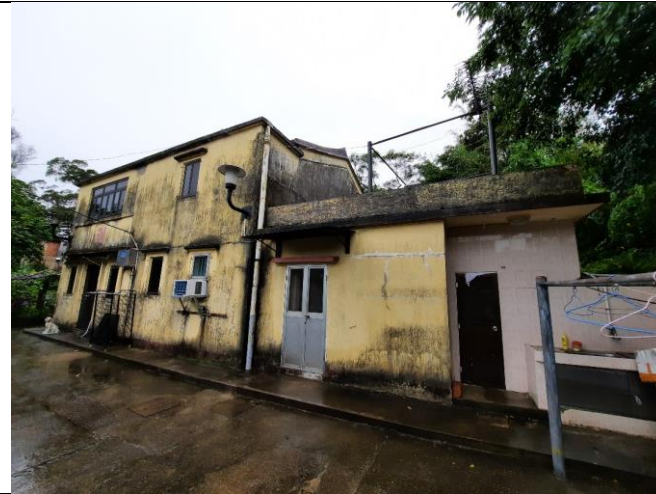
Photo 2: General View of NP-10
