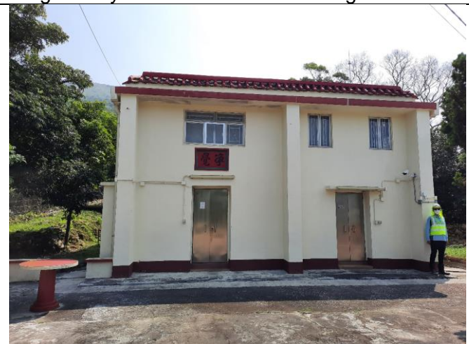
Photo 6: General View of NP-11
