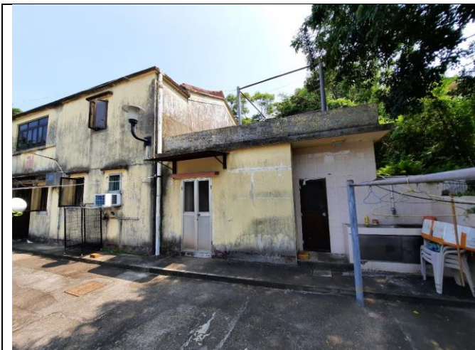
Photo 1: General View of NP-10
