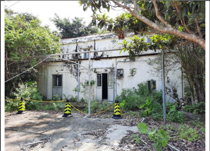
Photo 9: NP-19 has been fenced off in accordance to EM&A Manual.
