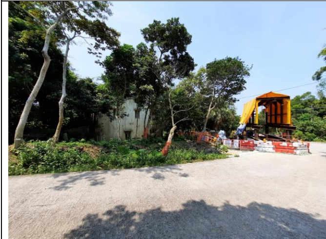
Photo 10: Construction works in close proximity of NP-19
