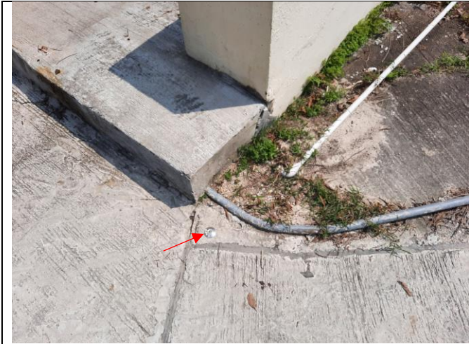
Photo 7: Ground settlement marker for settlement monitoring was installed at the entrance of NP-11.
