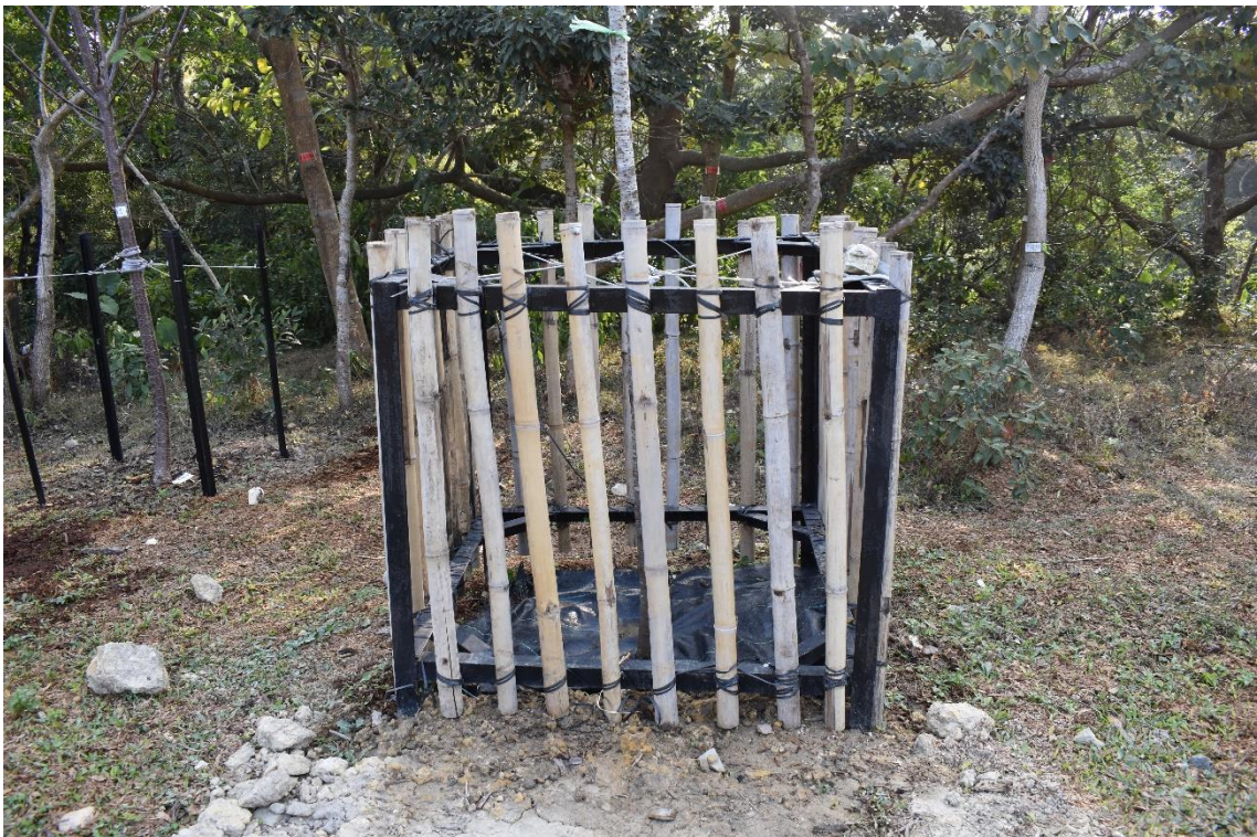
Appendix A.4.2: Sample Photo for Erection of Solid Fencing Around Plant Species
