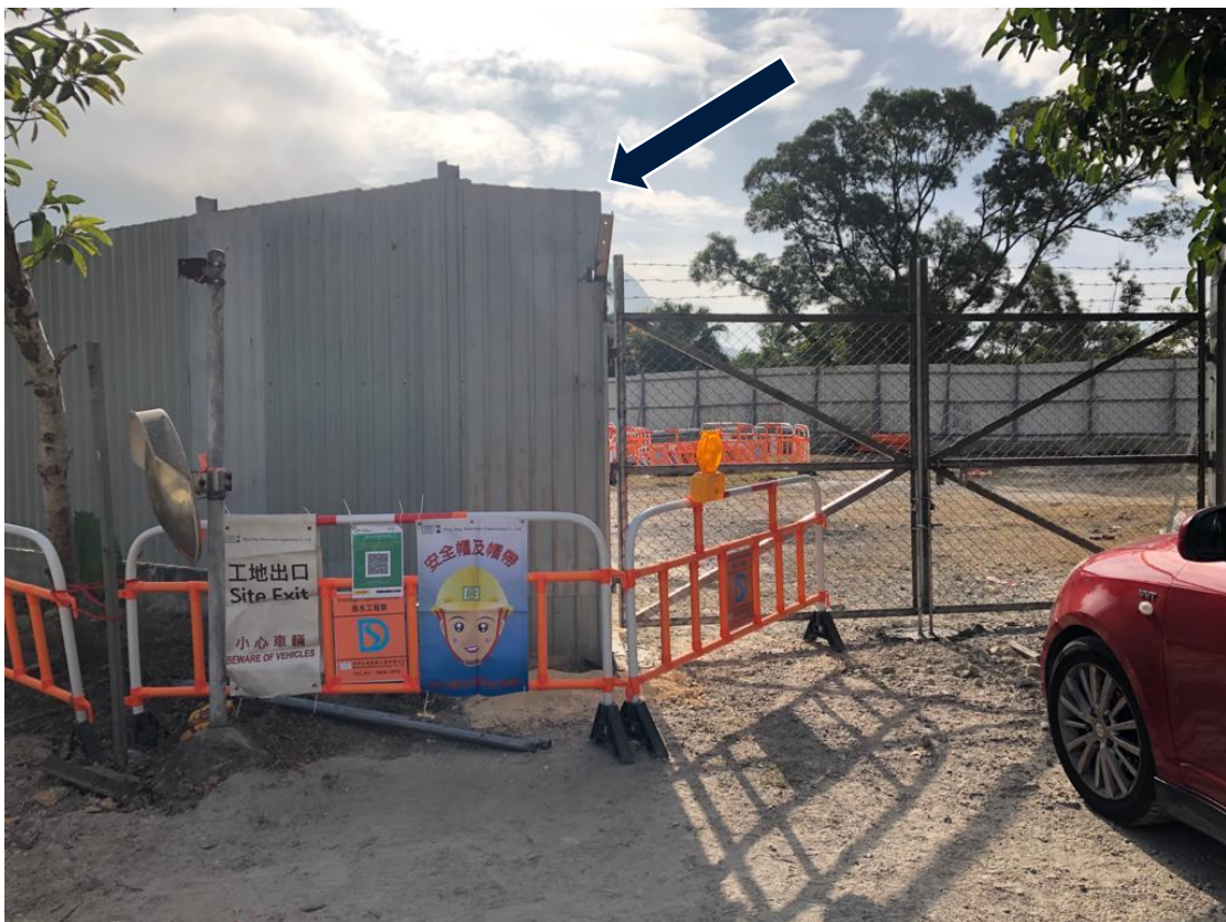
Appendix E2: Hoarding of the Site Office
