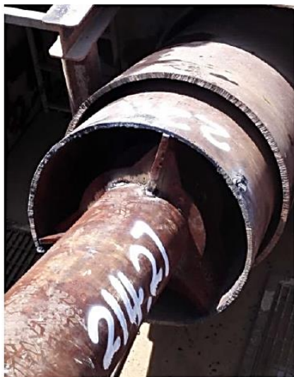
Photo of DN355mm casing installation
