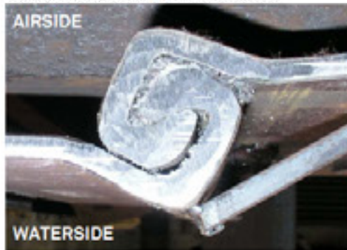
Figure 4: LARSEN-Sheet pile (Type 603)
