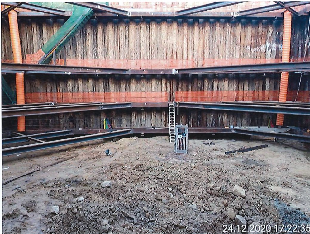
The plastic sealant application allowed the dewatering purpose inside the cofferdam
