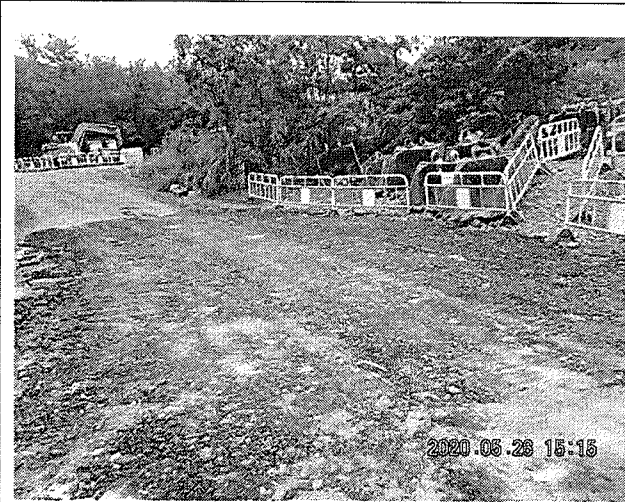
Photo 200526_001 (Near Work Shop) (Improved)
