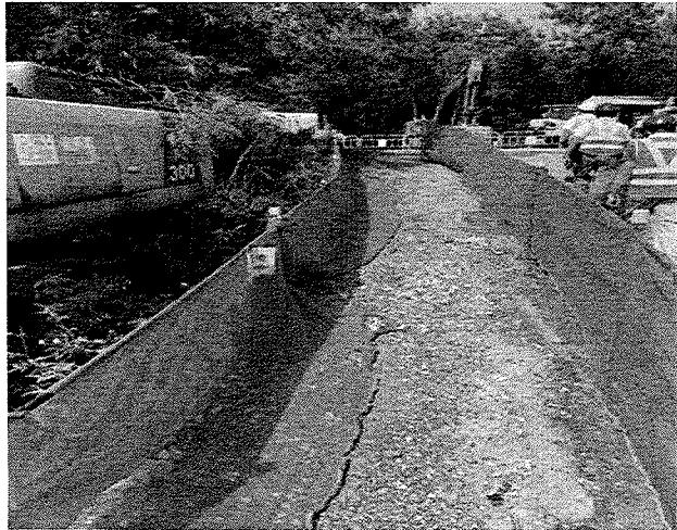
Photo 200820_001 (Near Workshop) (Improved)
