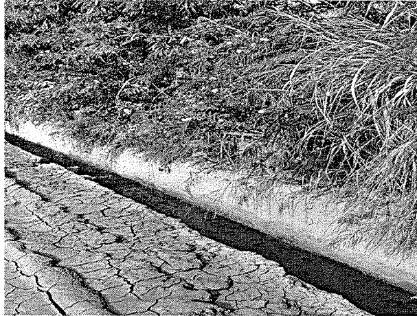
Photo 210331_001 (Near 3RS Platform) (Improved)
