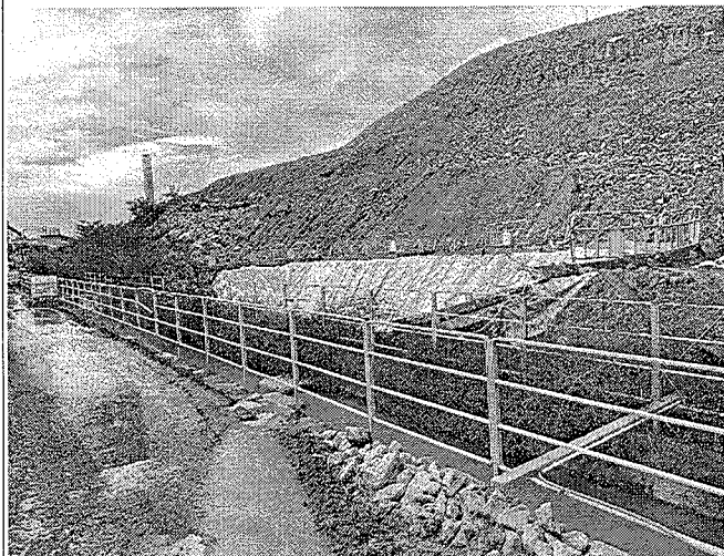
Photo 210923_001 (Near A3 pier)
