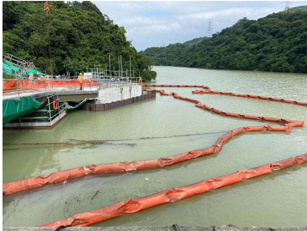
Figure 1 – Site Photo of KBR Works area taken on 19 October 2021
