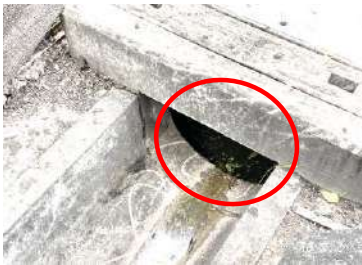
(Observed on 20 October 2023)
