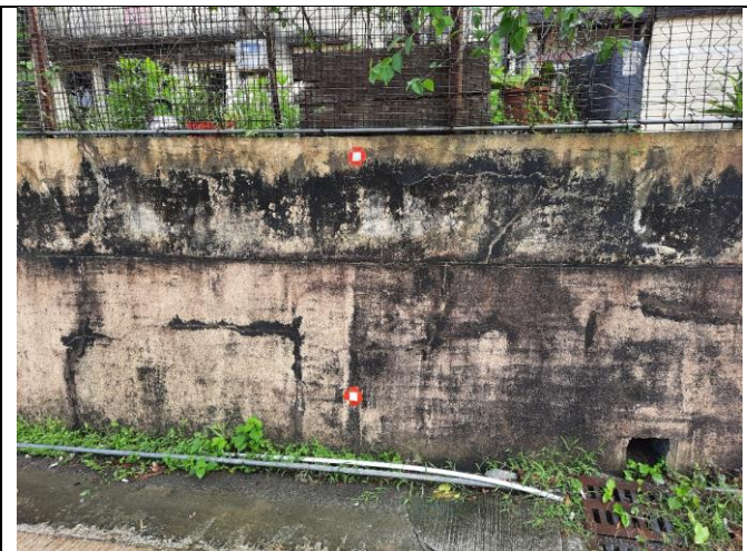
Photo 3: Additional reflective targets for settlement monitoring were installed on the fence wall at NP-10.
