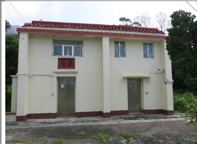
Photo 4: General View of NP-11
