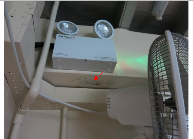
Photo 6: Tell-tale for crack monitoring was installed at NP-11.
