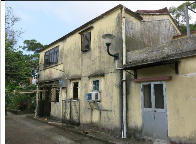
Photo 1: General View of NP-10
