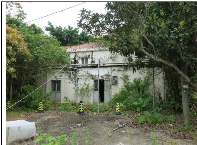
Photo 7: NP-19 has been fenced off in accordance to EM&A Manual.
