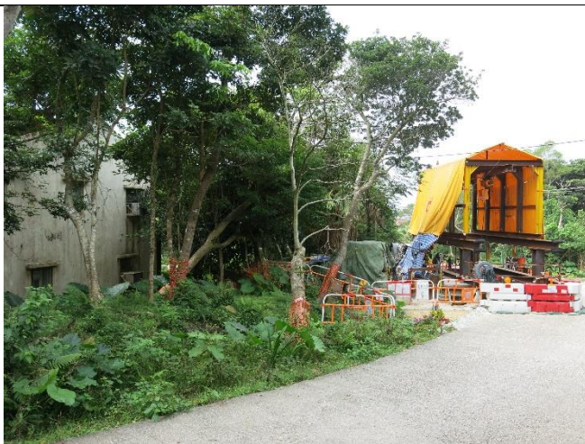
Photo 8: Construction works in close proximity of NP-19
