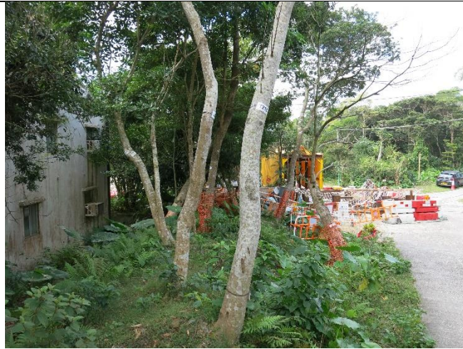
Photo 8: Construction works in close proximity of NP-19
