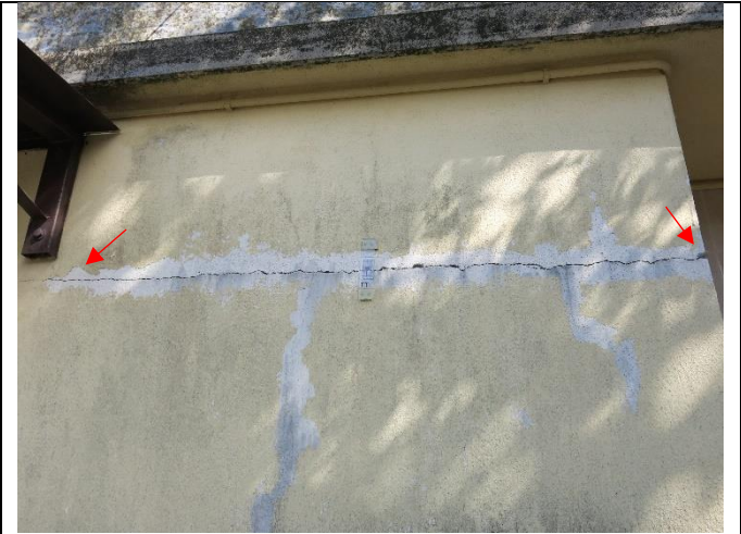
Photo 3: Tell-tales for crack monitoring were installed at NP-10.
