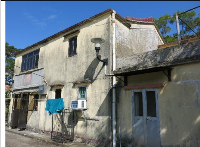
Photo 1: General View of NP-10
