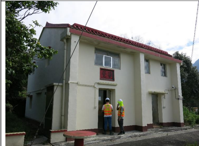
Photo 4: General View of NP-11
