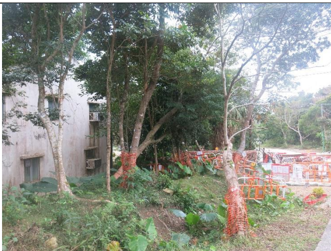
Photo 8: Construction works in close proximity of NP-19
