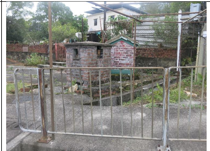
Photo 12: The notice at NP-26 was found missing. Replacement is required.
