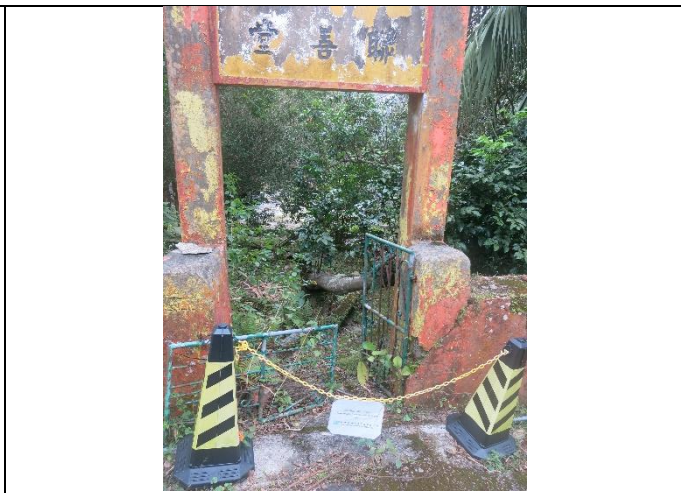
Photo 9: Access to NP-20 & NP-21 has been fenced off in accordance to EM&A Manual.
