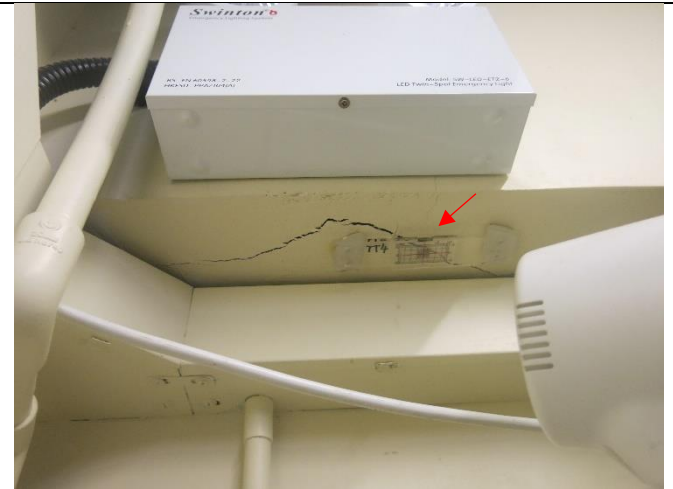
Photo 6: Tell-tale for crack monitoring was installed at NP-11.
