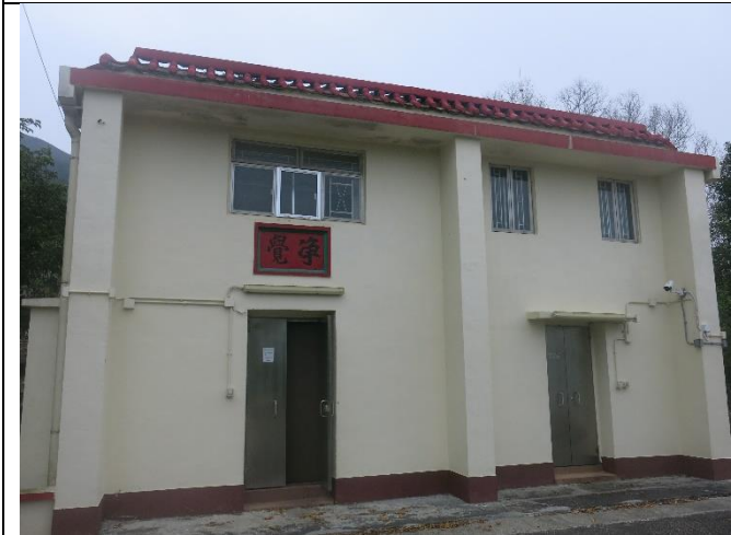
Photo 4: General View of NP-11
