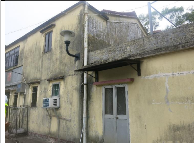
Photo 1: General View of NP-10
