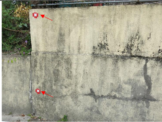
Photo 2: Reflective targets for settlement monitoring were installed on the fence wall at NP-10.
