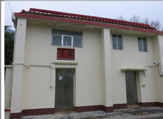
Photo 4: General View of NP-11
