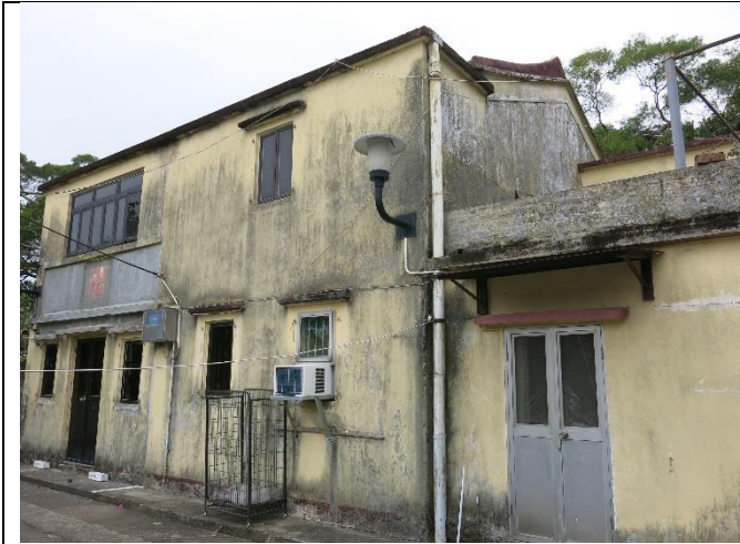
Photo 1: General View of NP-10
