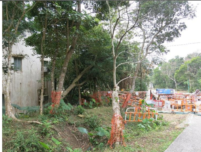
Photo 8: Construction works in close proximity of NP-19
