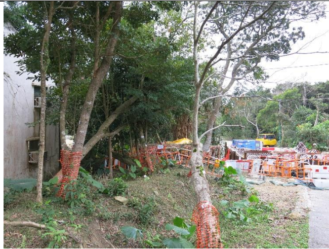
Photo 8: Construction works in close proximity of NP-19
