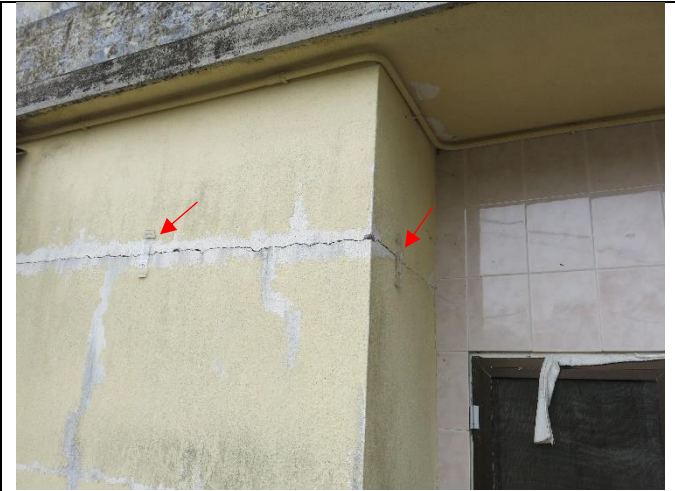
Photo 3: Tell-tales for crack monitoring were installed at NP-10.
