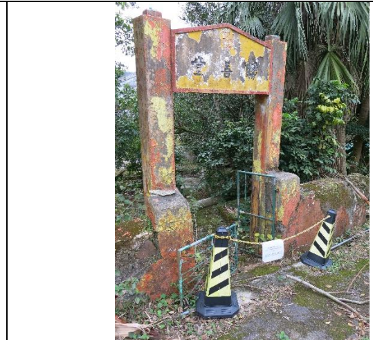
Photo 9: Access to NP-20 & NP-21 has been fenced off in accordance to EM&A Manual.
