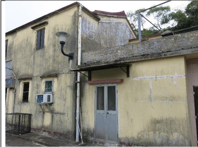
Photo 1: General View of NP-10
