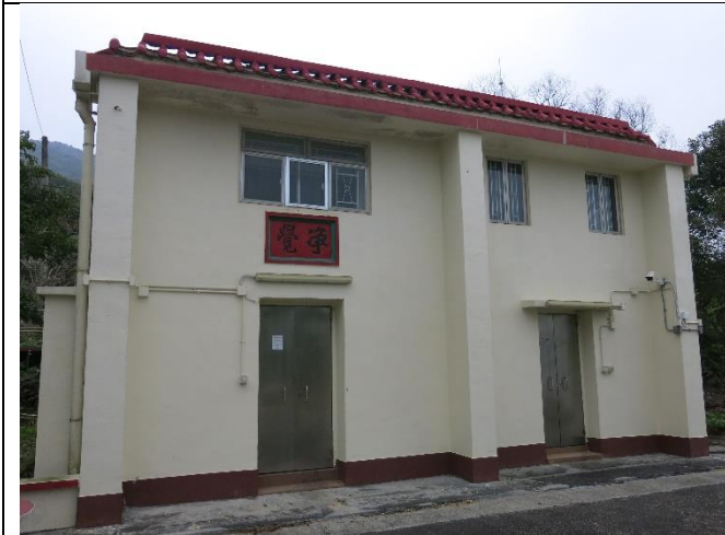
Photo 4: General View of NP-11
