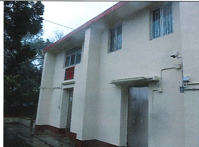
Photo 4: General View of NP-11
