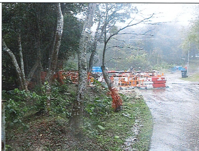
Photo 8: Construction works in close proximity of NP-19
