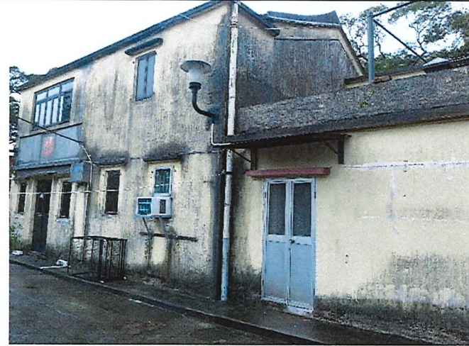
Photo 1: General View of NP-10
