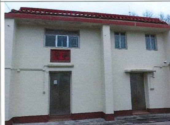
Photo 4: General View of NP-11
