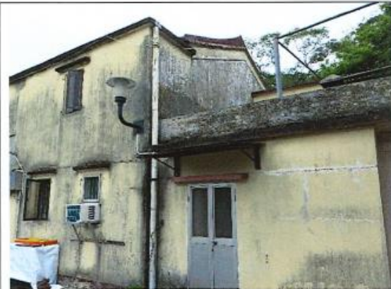
Photo 1: General View of NP-10
