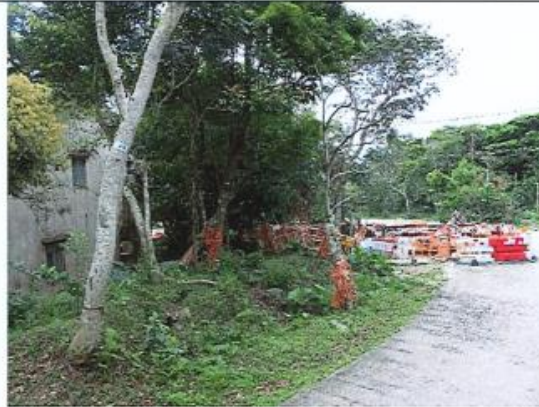
Photo 8: Construction works in close proximity of NP-19
