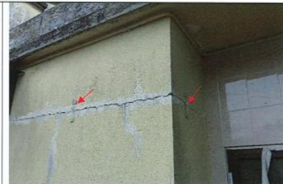
Photo 3: Tell-tales for crack monitoring were installed at NP-10.
