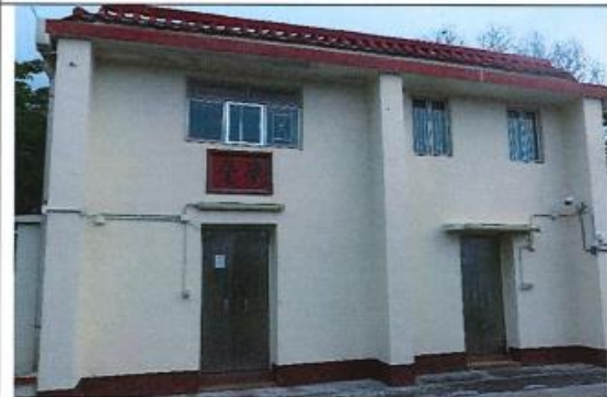
Photo 4: General View of NP-11
