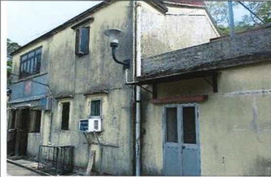
Photo 1: General View of NP-10
