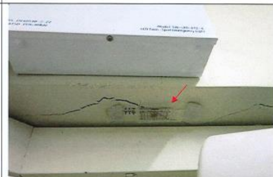
Photo 6: Tell-tale for crack monitoring was installed at NP-11.
