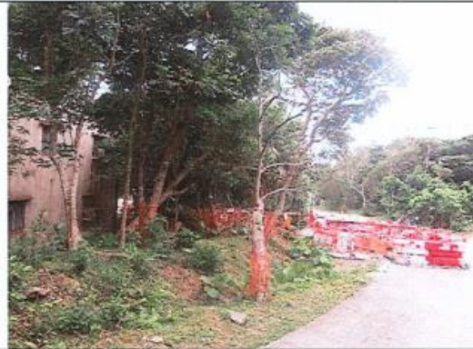
Photo 8: Construction works in close proximity of NP-19
