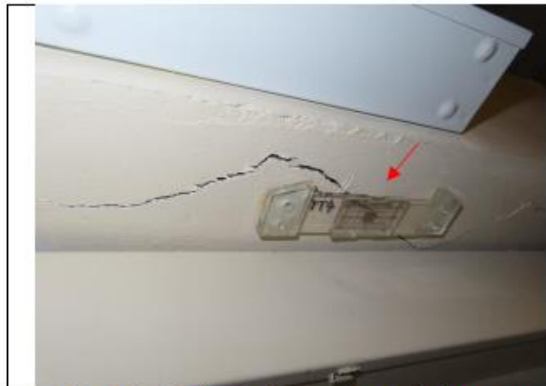
Photo 7: Tell-tale for crack monitoring was installed at NP-11.
