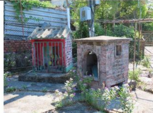
Photo 12: No temporary fence has been erected around NP-26 in mutual agreement with the villagers.
