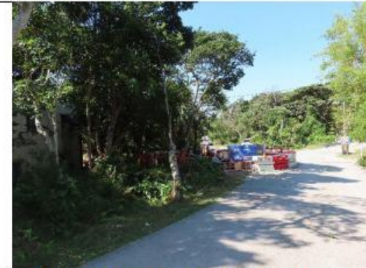
Photo 9: Construction works in close proximity of NP-19.
