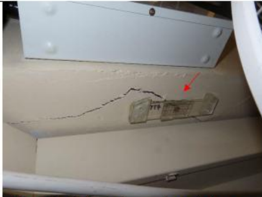
Photo 7: Tell-tale for crack monitoring was installed at NP-11.
