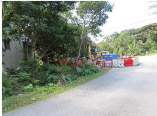
Photo 10: Construction works in close proximity of NP-19.
