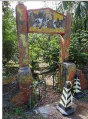
Photo 11: Access to NP-20 & NP-21 has been fenced off in accordance to EM&A Manual.
