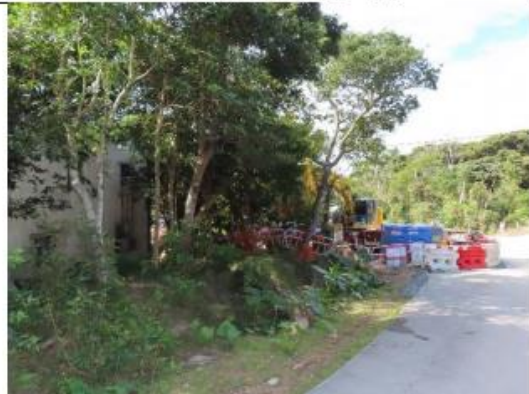
Photo 10: Construction works in close proximity of NP-19.
