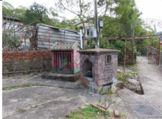
Photo 13: No temporary fence has been erected around NP-26 in mutual agreement with the villagers.
