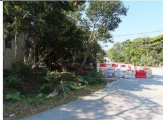
Photo 10: Construction works in close proximity of NP-19.
