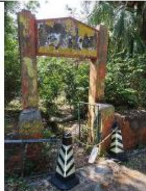
Photo 11: Access to NP-20 & NP-21 has been fenced off in accordance to EM&A Manual.
