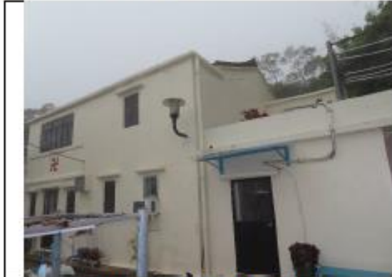
Photo 1: General View of NP-10
