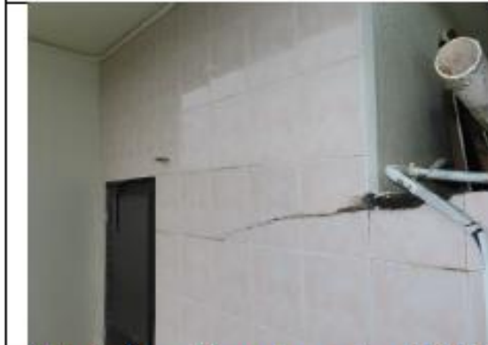
Photo 4: Renovation works were done at NP-10 except for the walls in Kitchen & Lavatory at the time of inspection.
