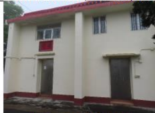
Photo 6: General View of NP-11
