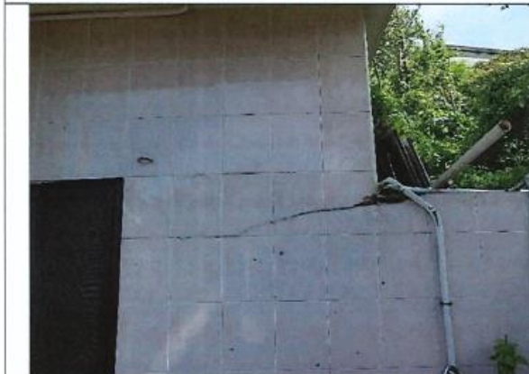
Photo 4: Renovation works were done at NP-10 except for the walls in Kitchen & Lavatory at the time of inspection.
