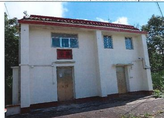
Photo 6: General View of NP-11
