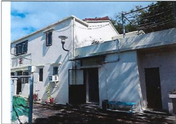
Photo 1: General View of NP-10
