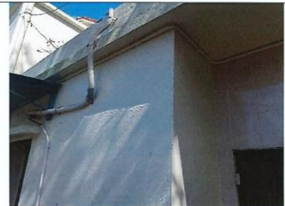
Photo 3: Tell-tales (TT1 & TT2) for crack monitoring were removed by the owner at NP-10 due to renovation works; Crack was repaired.
