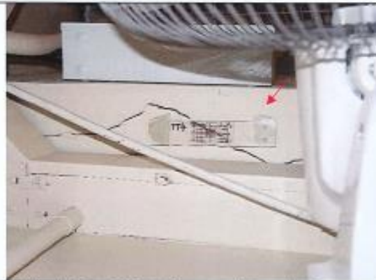
Photo 8: Tell-tale for crack monitoring was installed at NP-11.
