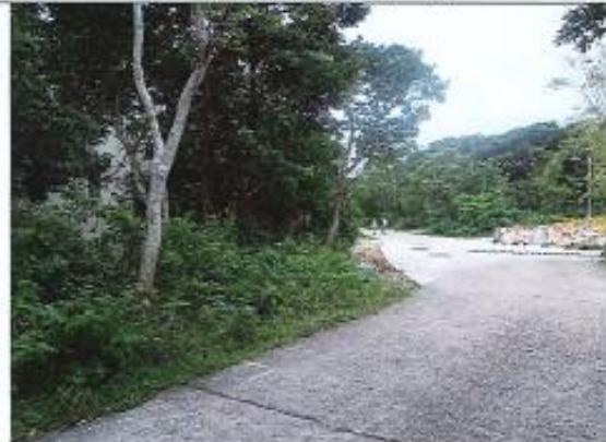
Photo 10: Construction works in close proximity of NP-19.
