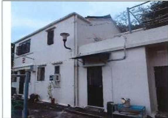
Photo 1: General View of NP-10
