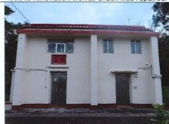
Photo 6: General View of NP-11
