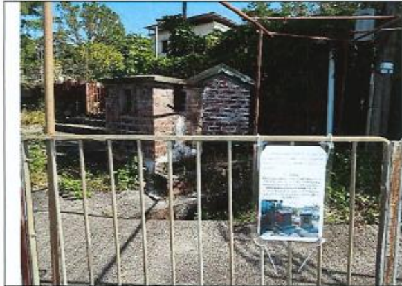
Photo 13: A warning notice was placed near NP-26.
