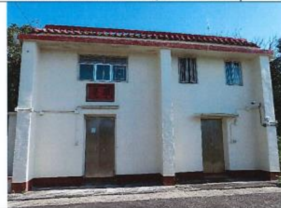
Photo 6: General View of NP-11
