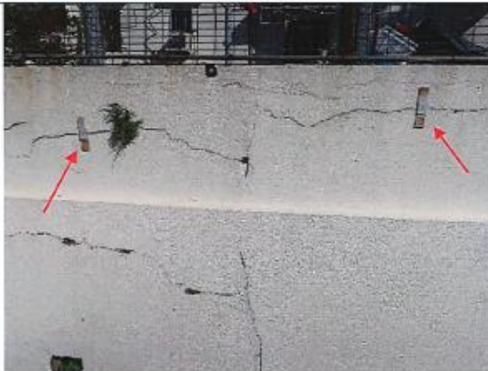
Photo 5: Tell-tales for crack monitoring were installed on the fence wall at NP-10.
