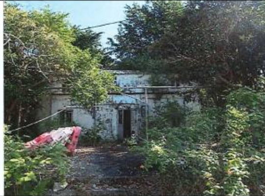
Photo 8: NP-19 has been fenced off in accordance to EM&A Manual.
