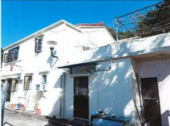
Photo 1: General View of NP-10
