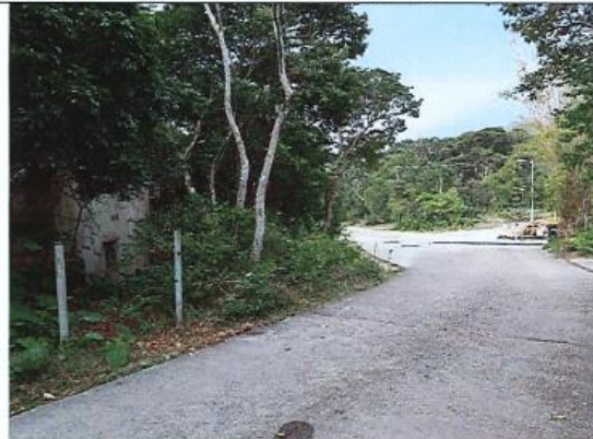
Photo 10: Construction works in close proximity of NP-19.
