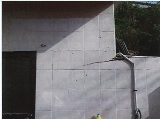
Photo 4: Renovation works were done at NP-10 except for the walls in Kitchen & Lavatory at the time of inspection.
