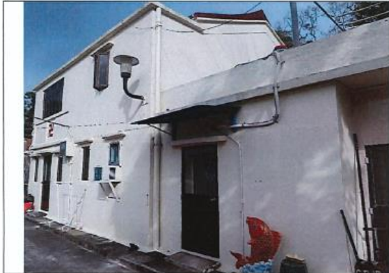
Photo 1: General View of NP-10
