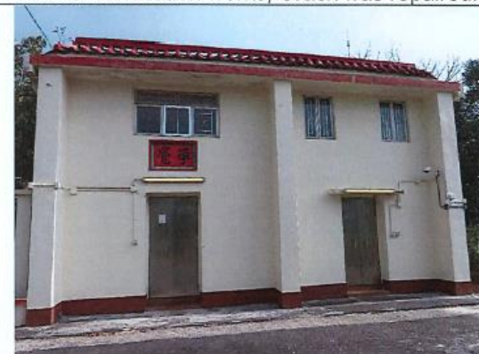
Photo 6: General View of NP-11
