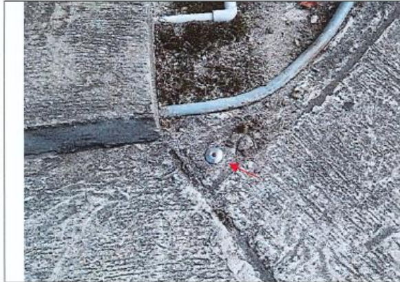
Photo 7: Ground settlement marker for settlement monitoring was installed at the entrance of NP-11.
