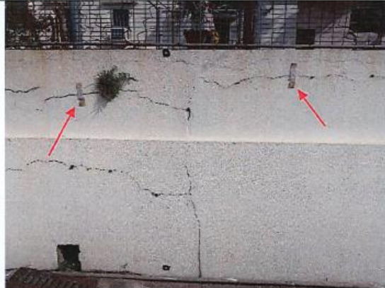
Photo 5: Tell-tales for crack monitoring were installed on the fence wall at NP-10.
