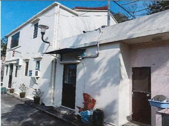
Photo 1: General View of NP-10
