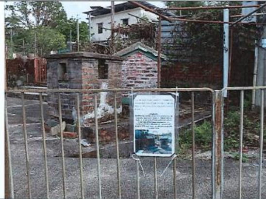
Photo 14: A warning notice was placed near NP-26.
