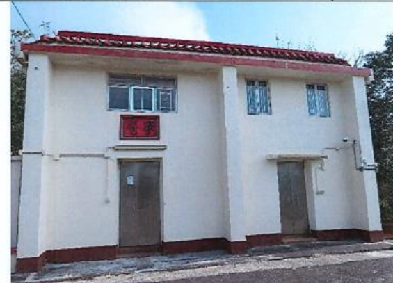
Photo 6: General View of NP-11
