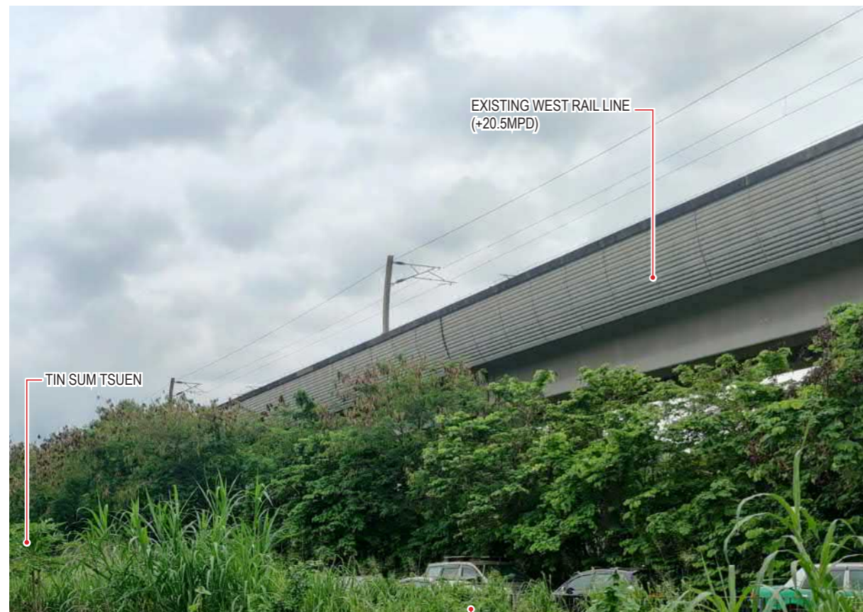
VSR1 - RESIDENTS IN TIN SAM TSUEN - EXISTING SITE CONDITION
