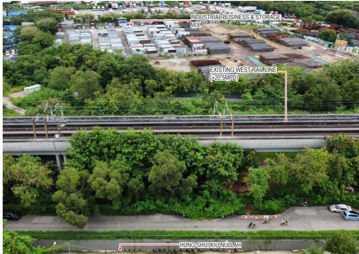
VSR3 - POTENTIAL RESIDENTS IN RESIDENTIAL SITES (AREAS 28B) UNDER HSK/HT NDA (+45MPD) - EXISTING SITE CONDITION
