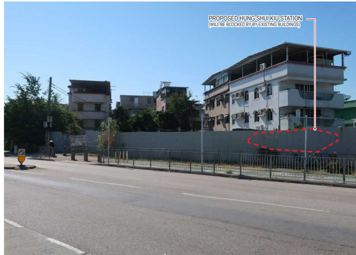
VSR2 - POTENTIAL RESIDENTS IN SAN LEE UK TSUEN (RETAINED VILLAGE UNDER HSK/HT NDA) -WITHOUT MITIGATION MEASURES
