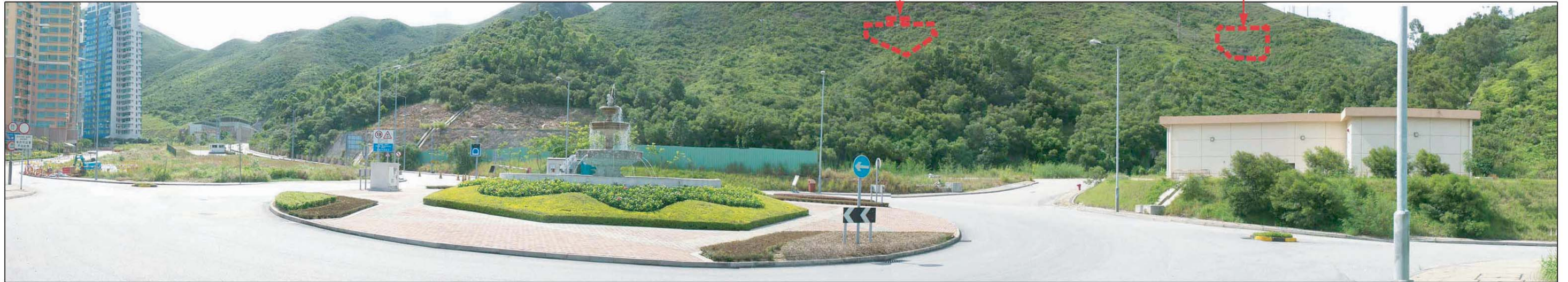
迴旋處景觀直望工地。 View from turning circle looking directly at the site.
